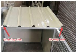
2. Place the next sheet to overlap the last sheet, ensuring the overlap side of the sheet is on top of the first sheet. Repeat with the third sheet and adjust the amount of overlap to centre the sheets on the kennel, ensuring equal overhang each side that the roof section is square with the kennel and there is 60mm overhang past the middle bearer.
