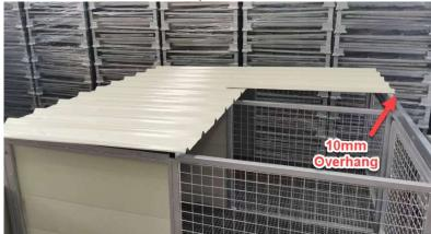
4. Ensure the front and rear sheets align and centre the sheets to have equal overhang each side, rechecking for a 10mm overhang on the front and being aligned through the sheet overlaps sections.
