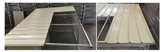
4. Ensure the front and rear sheets align and centre the sheets to have equal overhang each side, rechecking for a 10mm overhang on the front and being aligned through the sheet overlaps sections.
