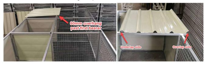
2. Place the next sheet to overlap the last sheet, ensuring the overlap side of the sheet is on top of the first sheet. Repeat with the 3<sup>rd</sup> and 4<sup>th</sup> sheet and adjust the amount of overlap to centre the sheets on the kennel, ensuring equal overhang each side. Also ensure the roof section is square with the kennel and there is 60mm overhang past the middle bearer.
